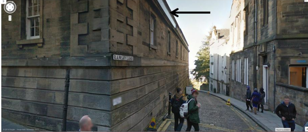
Fig. 3.26: Weaving Mill landmark at the top of Ramsay Lane, used as a navigation point by SpaceBook
